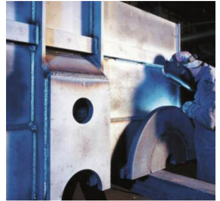
Heavy structure welding.
